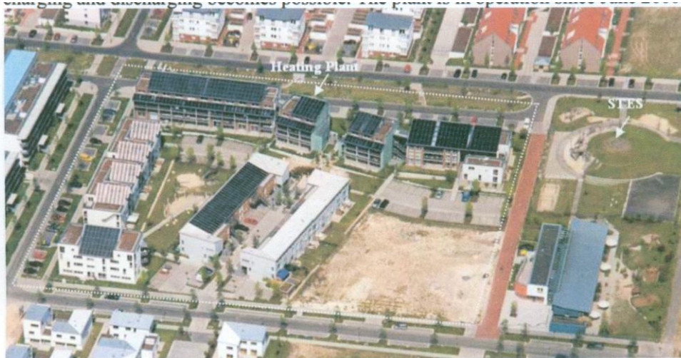
Fig. 2-30: CSHPSS in Hannover (source: Gockell)
