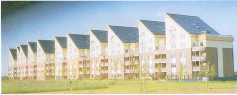
Fig. 2-29: Multifamily house with solar roof in Rostock
